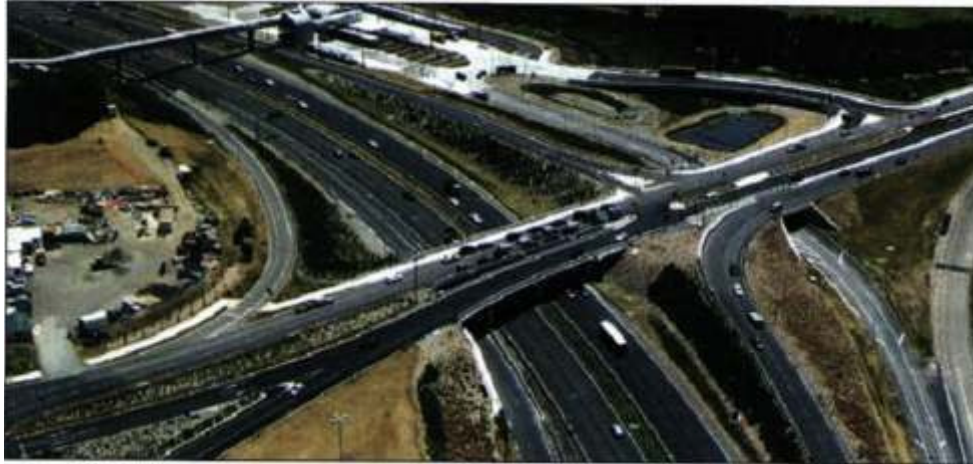
ESMONDE INTERCHANGE. AUCKLAND
